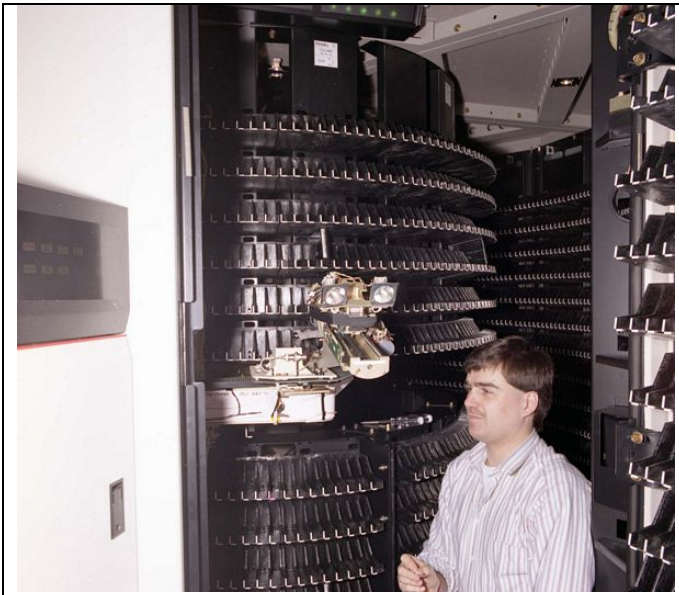
The scale of the silo is difficult to grasp from the numbers but it dwarfs whoever is working on it.
