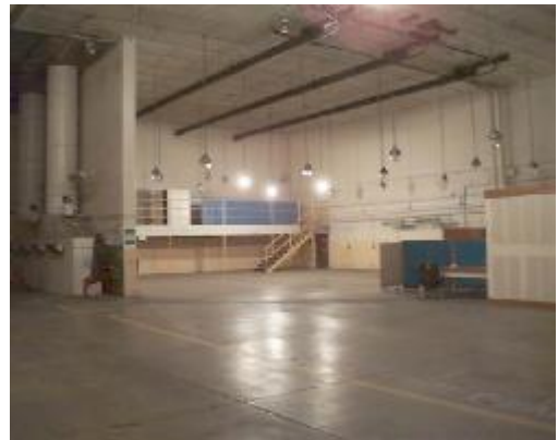
Cavernous interior of Building 45 (40 foot ceilings!)
