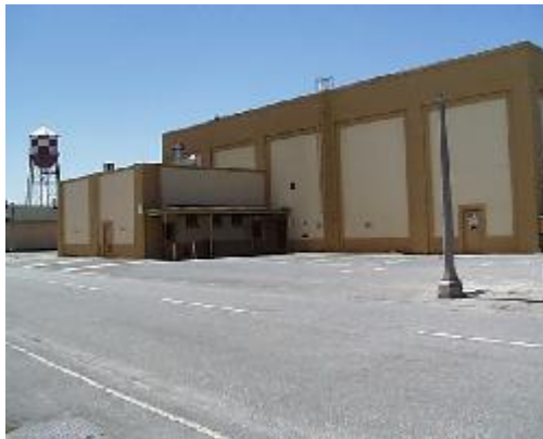
New Storage Area - Building 45 Visible Storage (Bldg 126) is across from the water tower
